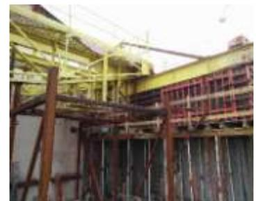
Fig. 11 Construction of a new supporting wall for a historic gantry, own archive, 09.03.2016
