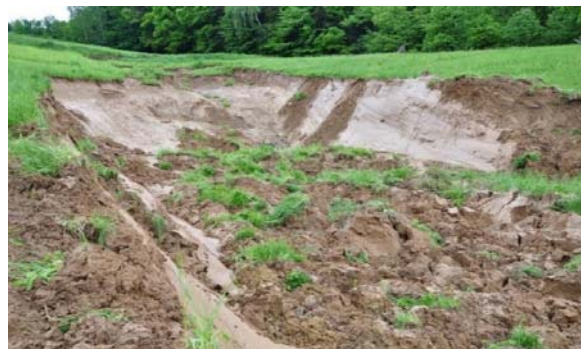
Photo 1. Landslide, Podkarpackie voivodeship, Strzyżów district; source: Archive of the Starostwo Office in Strzyżów
